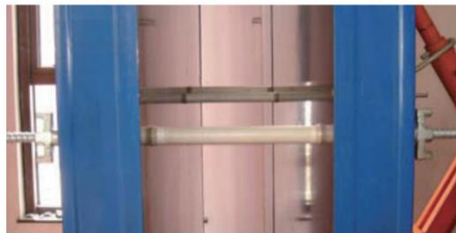
Convenient tie arrangement with the hole in frame
